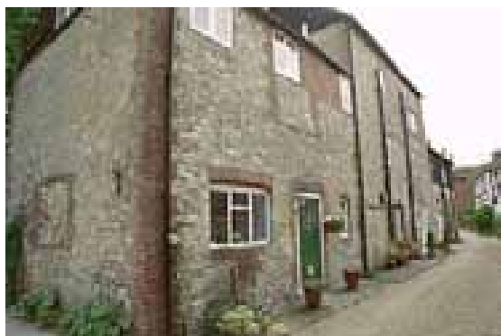
10-14 Brewers Yard, Storrington (above). Malthouse converted into five dwellings. Early C19.
