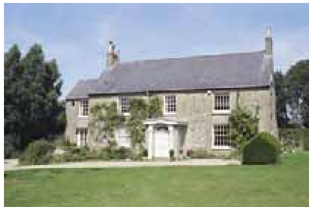
Hurston Place Farmhouse, Hurston Lane, Storrington (above).
