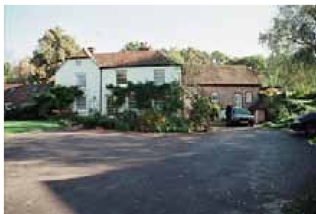
Chantry Mill, Sullington Lane, Sullington (above). L-shaped block comprising the mill and mill-house. Both C18.
